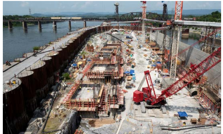
Framing Monoliths at Chickamauga Lock
