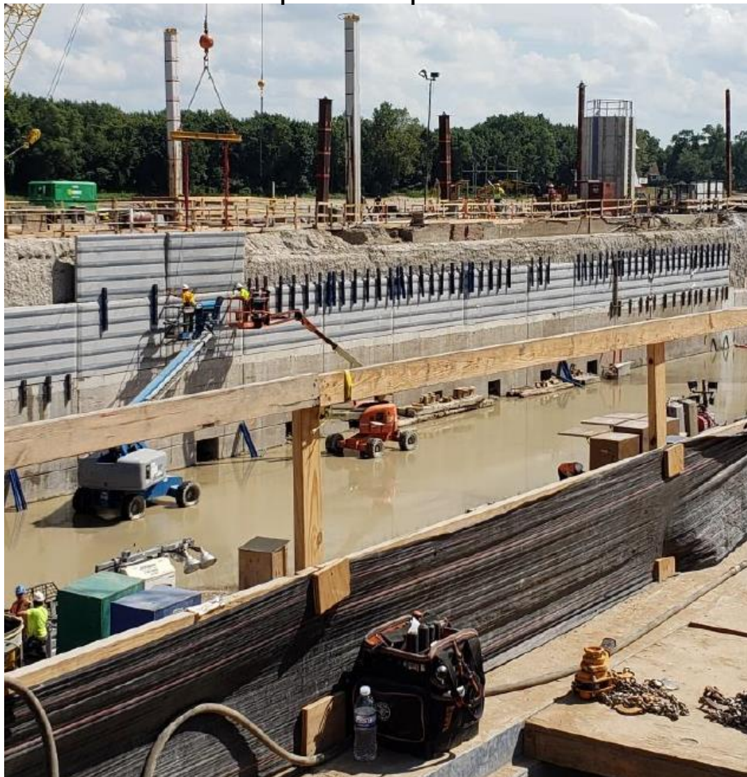
Vertical concrete pre-cast panel installation
