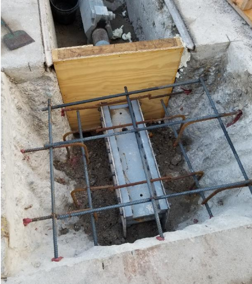
Miter gate anchorage repairs
