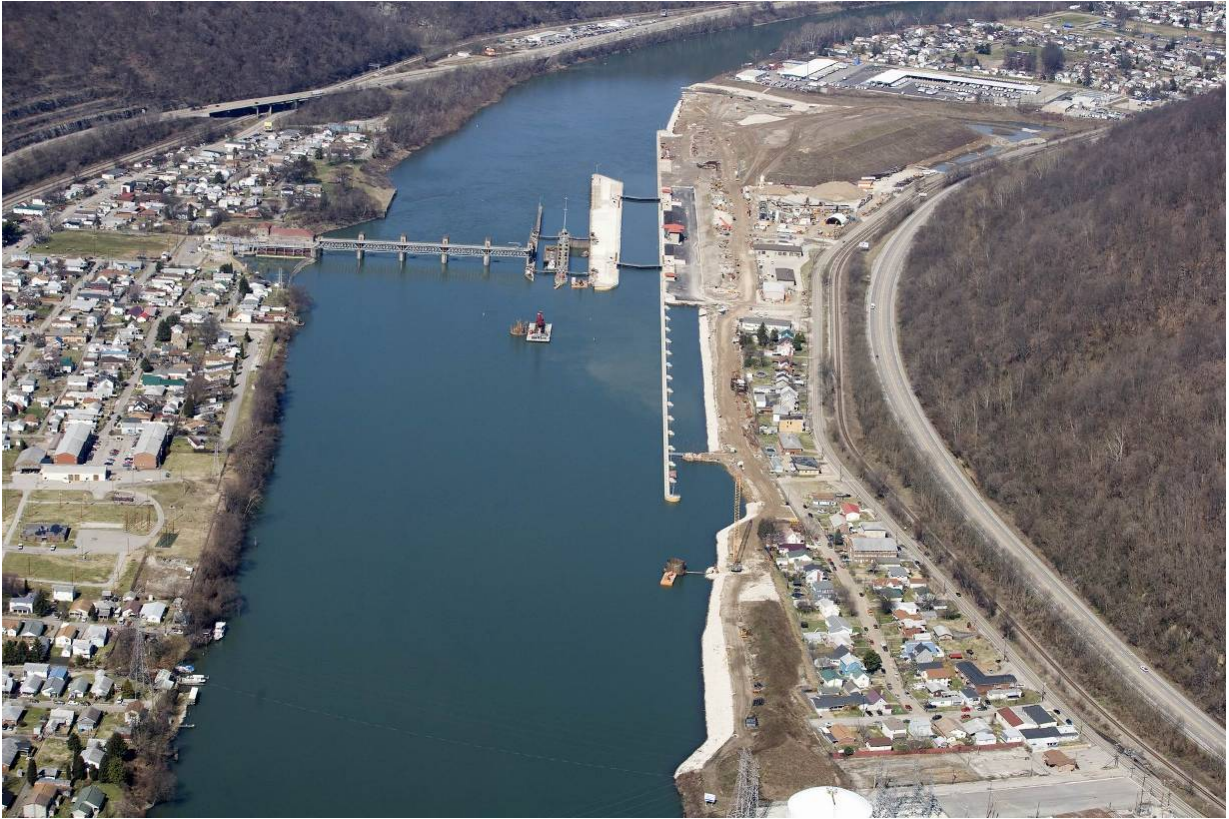
Figure 1 Photo: Marmet Locks & Dam
