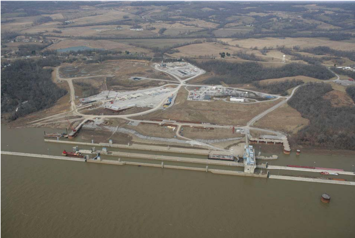
Figure 11 Olmsted Locks Progress Photo without Dam
