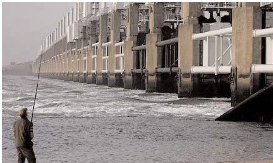
The Netherlands' Delta Works holds back North Sea surges.
