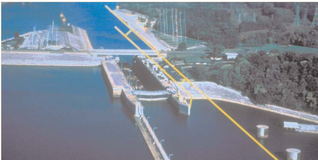
Kentucky Lock Funded. This is an aerial view of Kentucky Lock, looking downstream and showing the location of the lock addition in yellow. The President's budget did not request funds for the project, but the House appropriations bill includes $21.75 million for construction.
