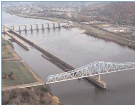
Hannibal Locks and Dam, looking upstream.
